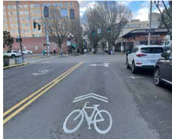
Shared lane with sharrow marking
